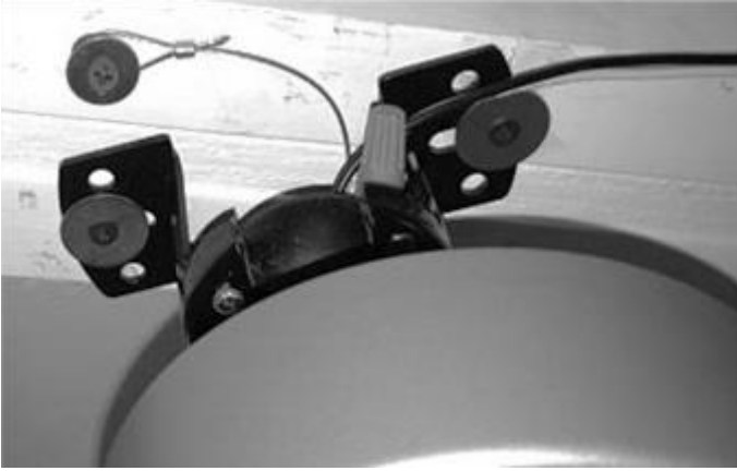
Photo 8: Safety cable attached near hanger
