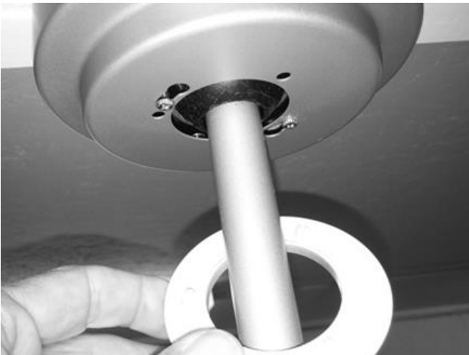
Photo 10: Key holes on the bottom of the canopy.
